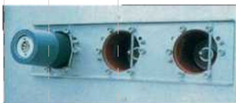
Fig.1 母线型套管座 busbar connecting bushing socket
