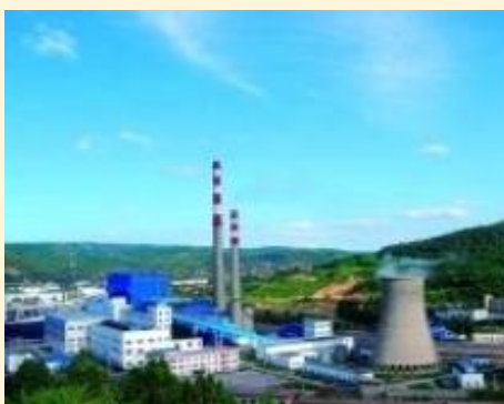
陕西神木电厂 2×660MW
