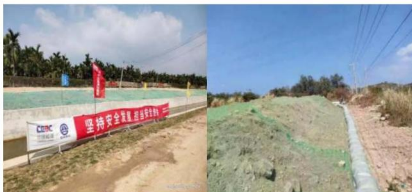
渠道边坡临时苫盖
