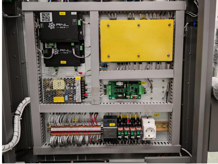
3-9 Check the dust accumulation of the cabinets regularly
