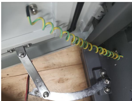
3-3 Check whether the nut of grounding stud is loose
