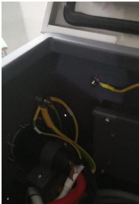
3-3 Check whether the nut of grounding stud is loose
