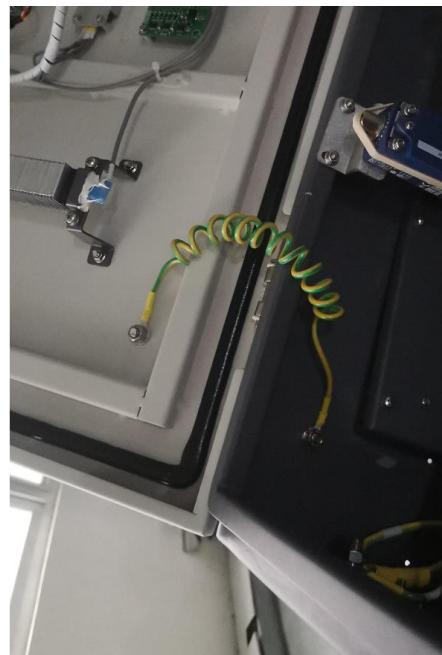
3-3 Check whether the nut of grounding stud is loose
