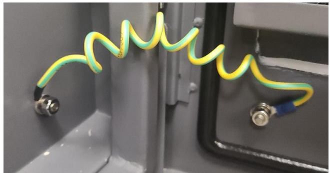
3-3 Check whether the nut of grounding stud is loose
