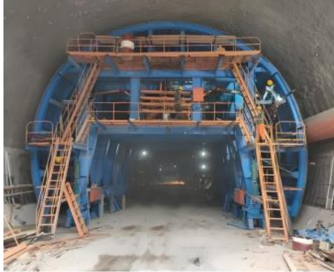
The tunnel layer distributor is used in conjunction with the lining trolley
