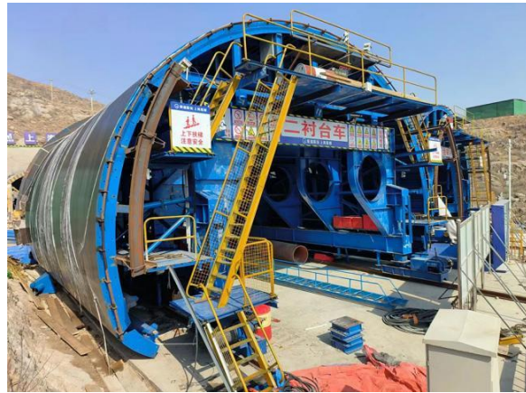
The tunnel layer distributor is used in conjunction with the lining trolley
