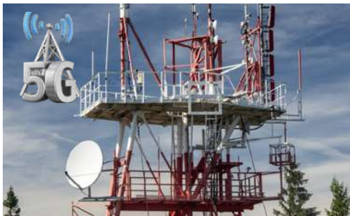
户外移动通讯基站智能电源解决方案 Solution for Telecommunication Station Power
