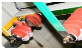
Fig. 5.1A Surge Arrester of Phase A Failure
