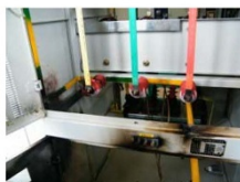
Fig. 5.1B The Phase to Phase Busbar Fault
