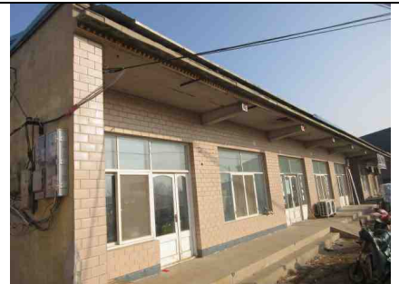
27) Outlook of factory building at another site
