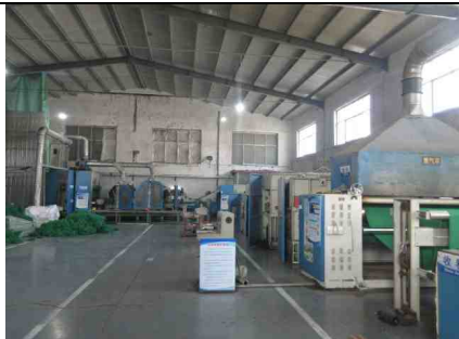
22) Another workshop for front processing (polyester fiber loosing, mixing, carding and weaving)
