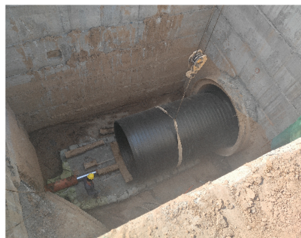
DN2000 Sewage Water Pipe Line Crossing under the Railway
