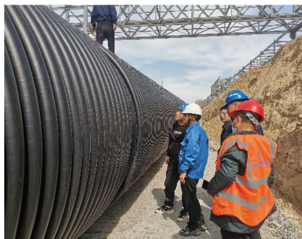
DN2500 Stormwater Line of Utilities
