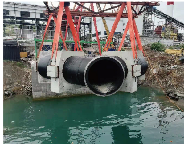
DN2200 Tee of Marine Intake Pipe Line
