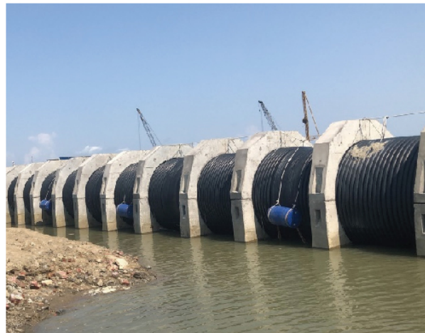
Marine Intake/Outfall Pipe Line
